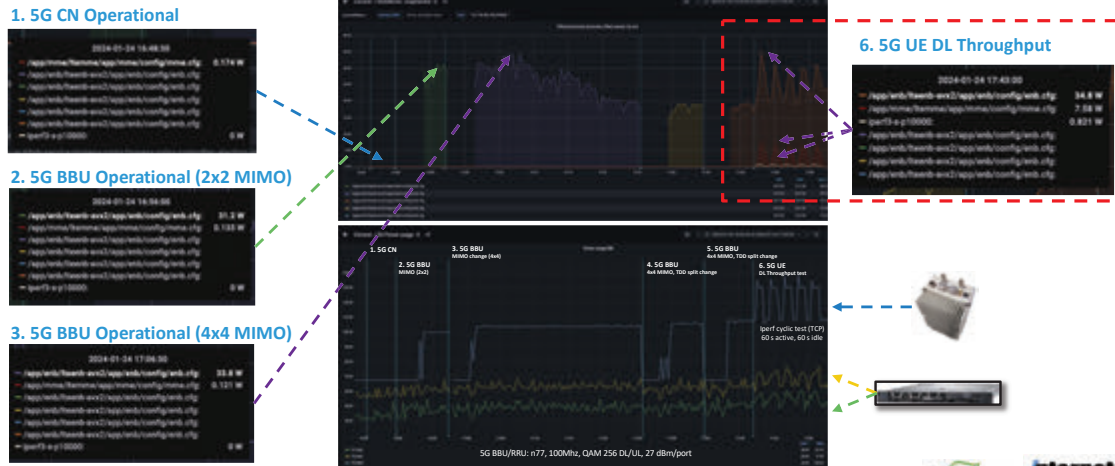
Page 31 | © 2024 INTERNET INSTITUTE. All Rights Reserved. Source ININ: Power Usage - Process Level
